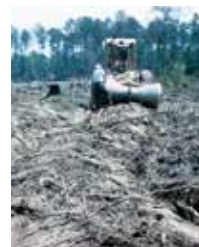
Bedding plow with compacting roller used to raise the soil in a planting row.
